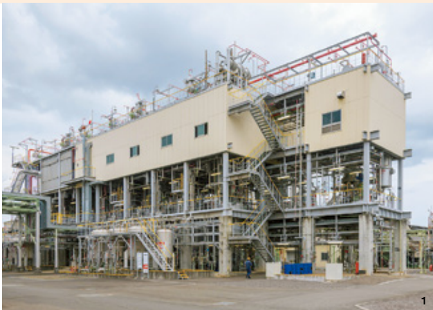
1. Sumisoya production plant. The top floor is walled to ensure a controlled environment for input of raw materials. 2. Reactor for synthesizing the compound.
