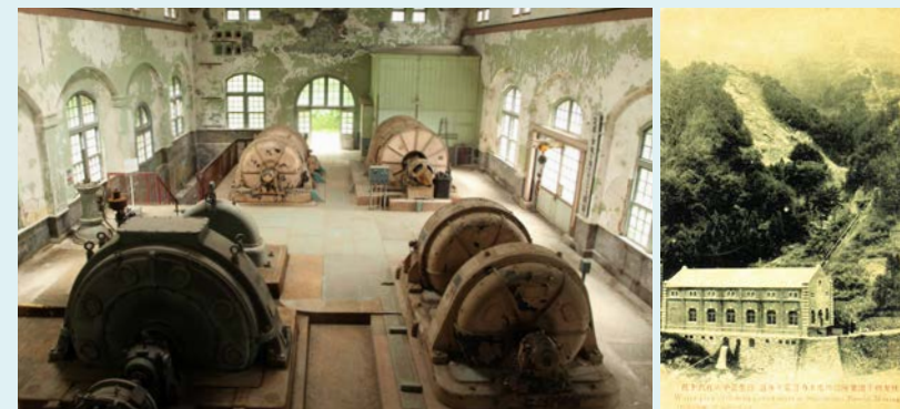
Interior of the former Hadeba Power Plant in Niihama, which remains to this day (photo above, courtesy of Niihama City). One of the original German power generators (front left) and three Japanese frequency converters are shown. Preparations are underway to open the plant to the public as a registered tangible cultural property of Japan. The plant, completed in 1912, had a water drop of 597 meters (photo right), the highest in Asia at the time.
