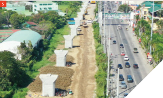
Progress of the North-South Commuter Railway Project in the Philippines 3 . Sumitomo Mitsui Construction is in charge of three station buildings, which will be constructed near the former station buildings of the Philippine National Railways. 4 . From the fabrication yard, 4,511 precast segments will be trucked to the site and erected step by step. 5 . 347 piers will be constructed.
